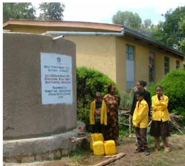
School Rainwater harvesting in Ethiopia. © UN-Habitat
